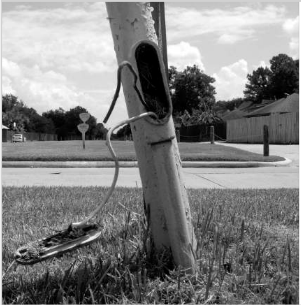
Fig. 9–29. Damaged cathodic test station (Courtesy Miesner, LLC)
