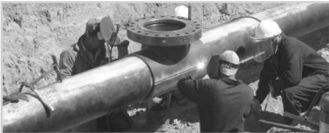
Fig. 9–24. Welding a hot tap fitting onto the line (Photo by Frank Gonzales)
