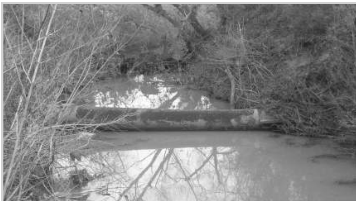
Fig. 9–7. Natural gas pipeline exposed in a drainage ditch (Courtesy Miesner, LLC)
