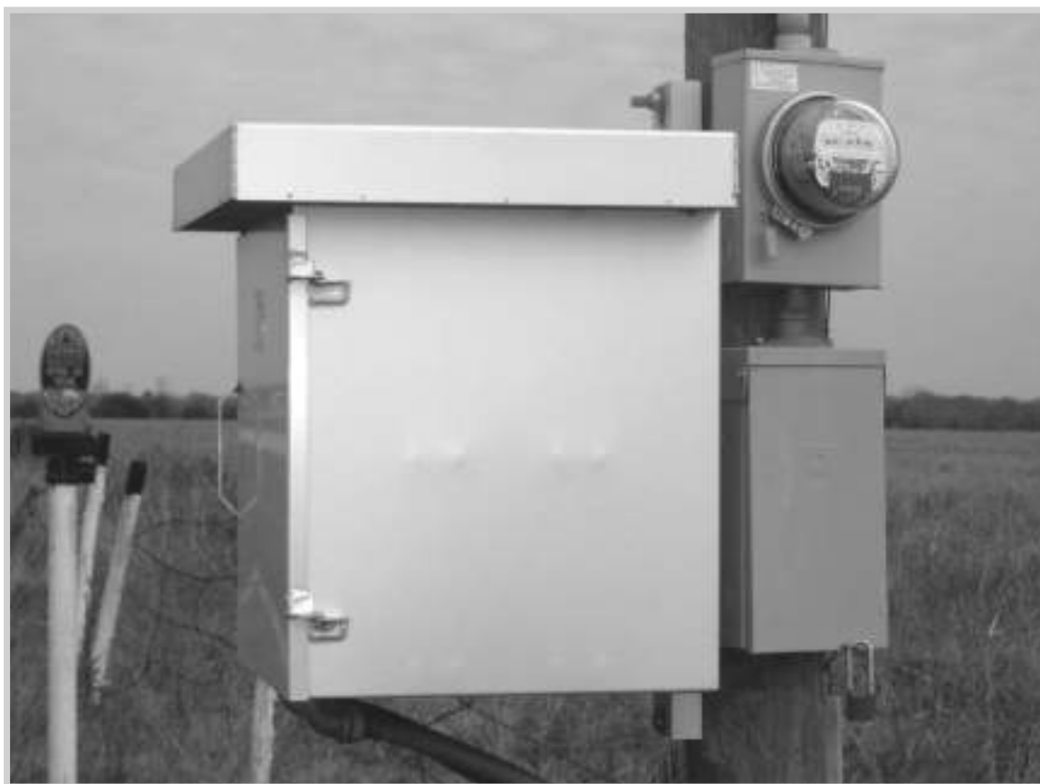
Fig. 9–13. Pipeline rectifier. Note the power meter and breaker box on the pole next to the rectifier and the line markers in the background. (Courtesy Miesner, LLC)
