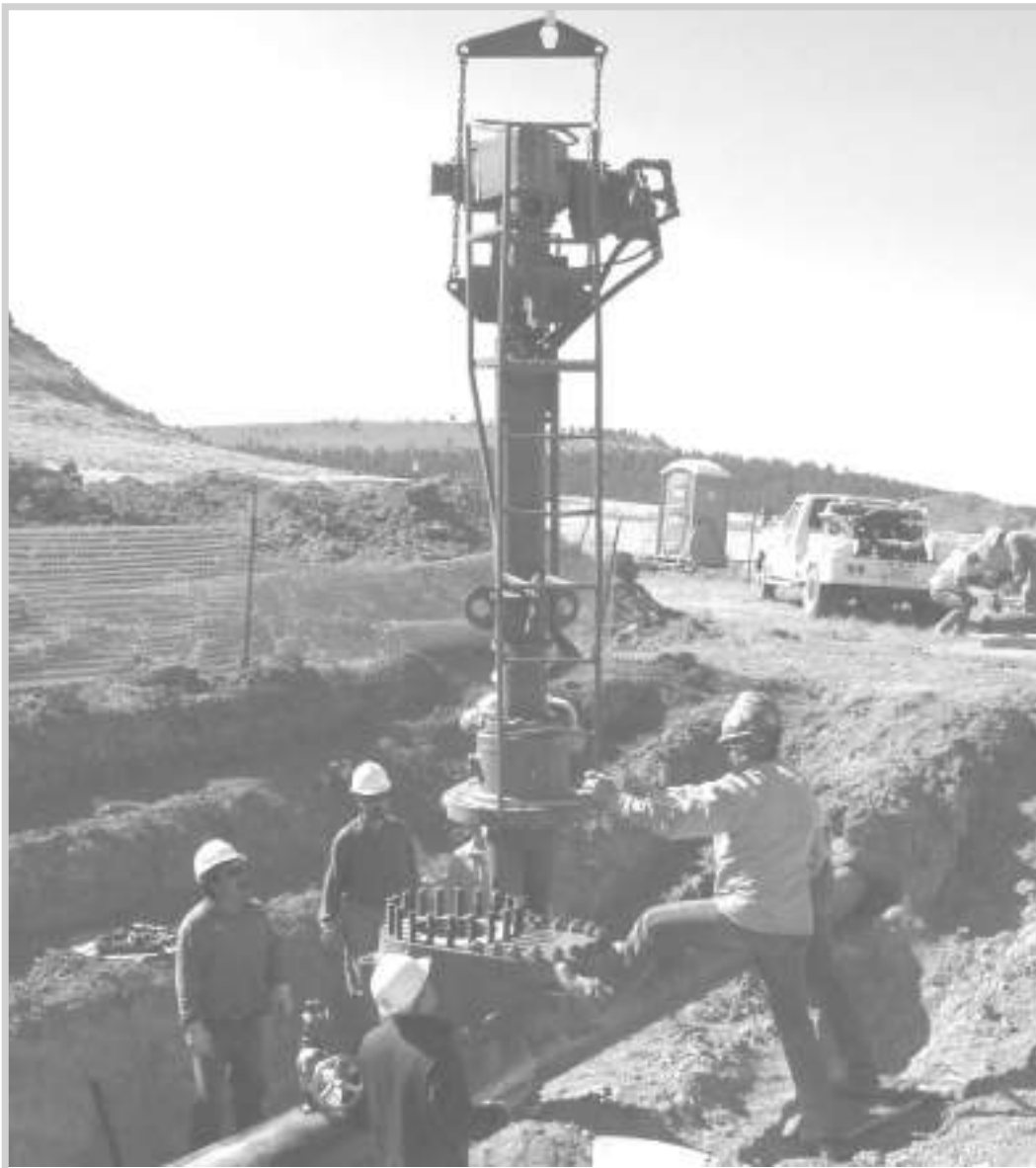
Fig. 9–25. Lowering the tapping machine. Note the valve is already bolted to the hot tap fitting. (Photo by Frank Gonzales)
