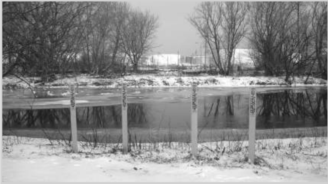
Fig. 9–10. Cleared and marked ROW (Courtesy Miesner, LLC)
