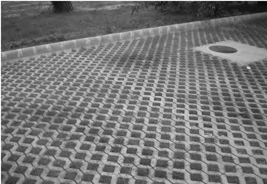
16-3. Pervious Paving System in Central Hungary
